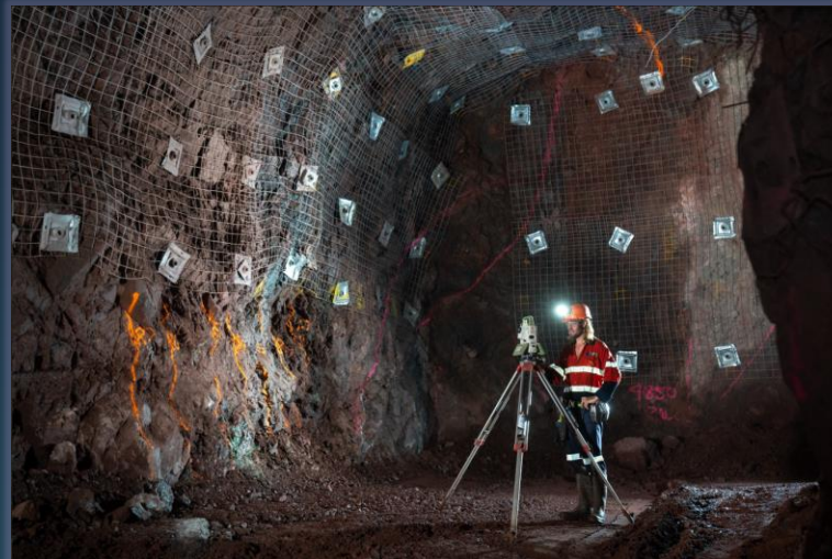
Established underground development
