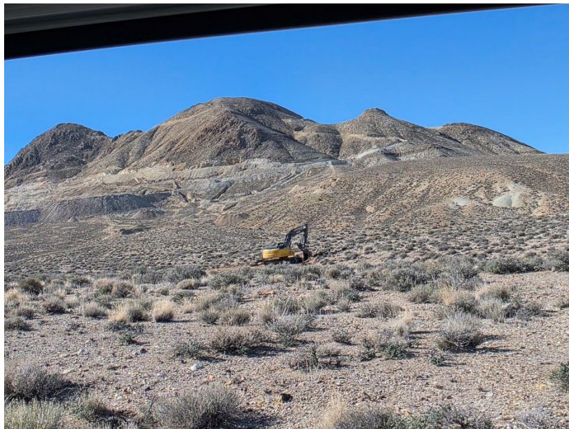
Figure 2: Drill Pad Construction
