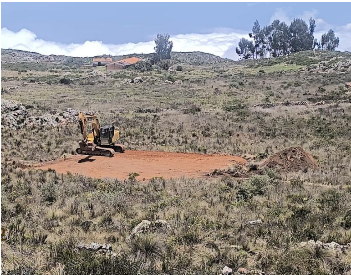
Figure 3. Drill pads at Flint
