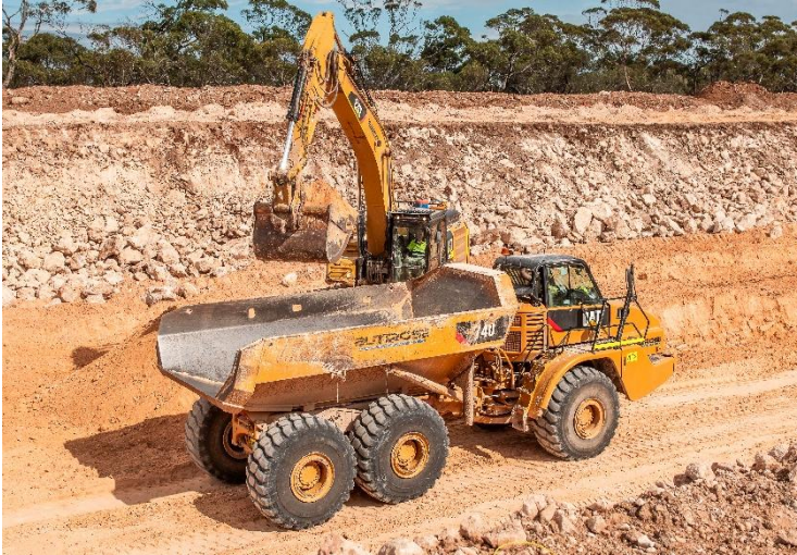
Excavation of the stormwater pond
