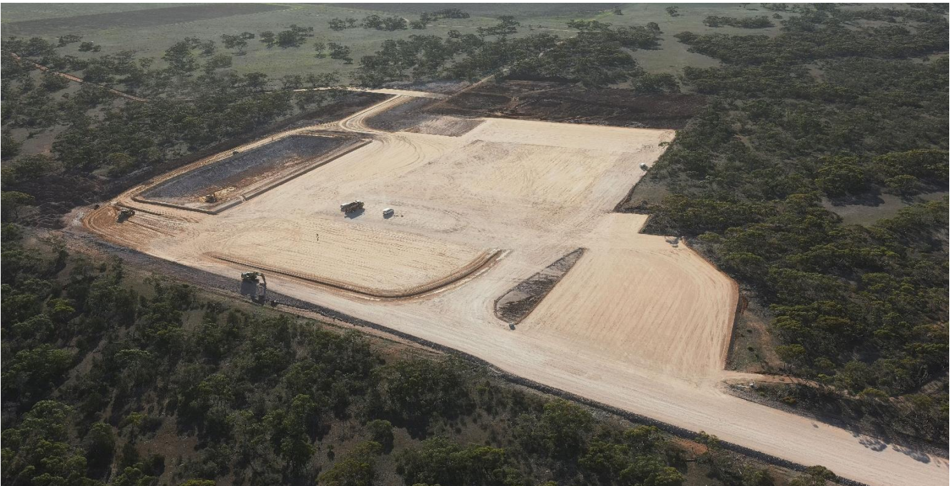
Processing Plant Pad Early Works Construction Completed
