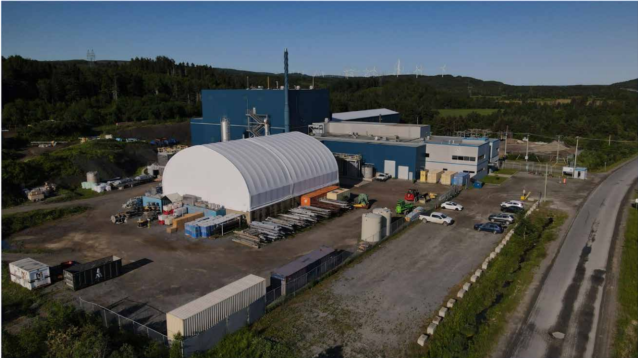
Figure 2.3: Aerial View of the Cap-Chat Plant
