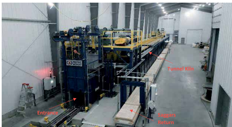
Figure 18. Tunnel Kiln in testing. (Source: AEM)
