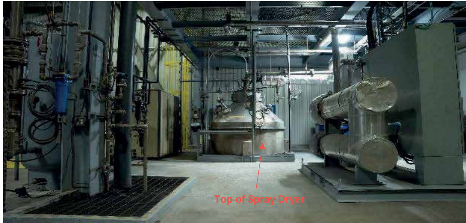
Figure 23. Spray Dryer. (Source: AEM)
