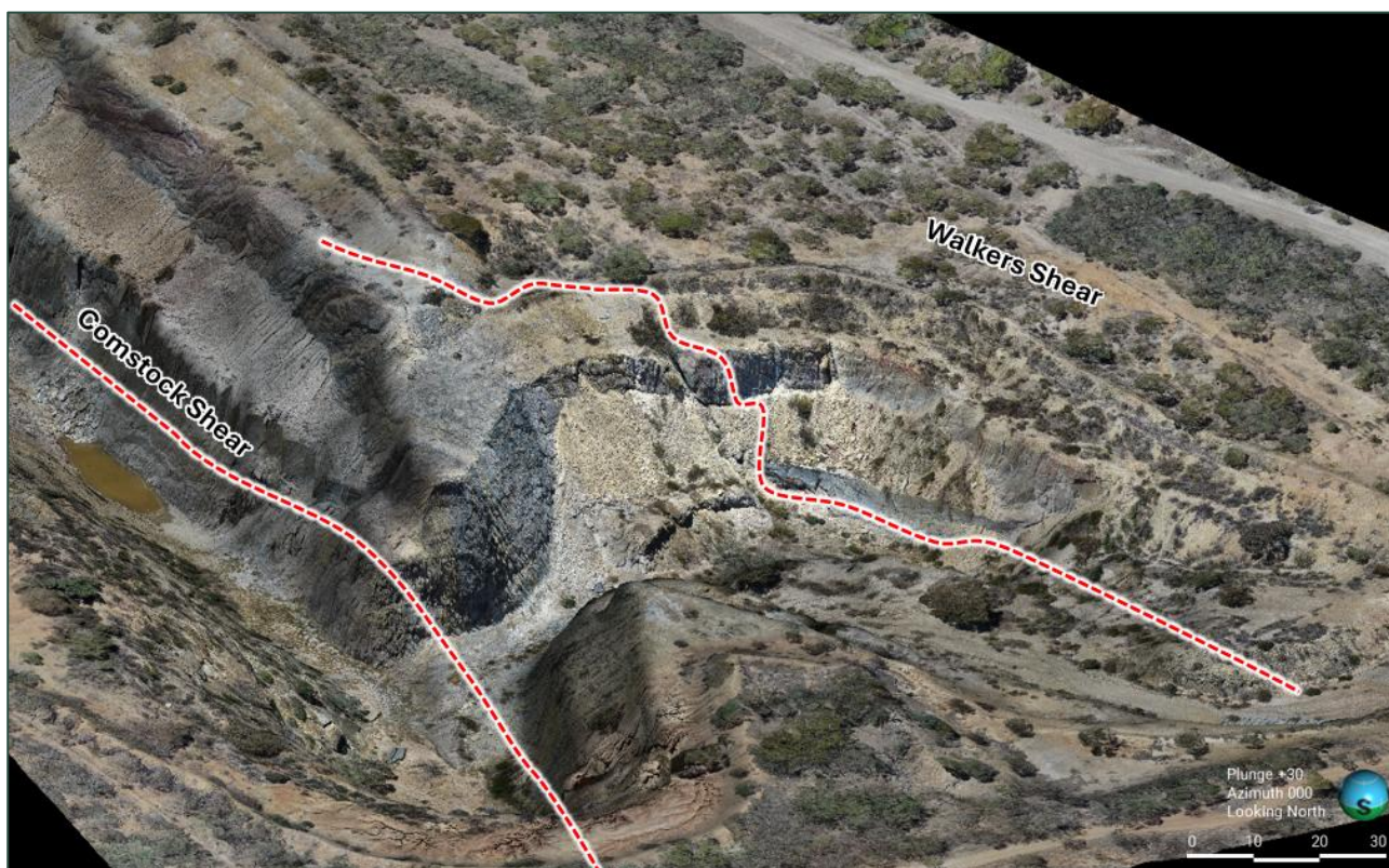
Figure 10: Comstock - View of the high-accuracy LiDAR and photogrammetry of the southern end of the Comstock open-cut with key projected structures – looking towards the North (azimuth 000) 26
