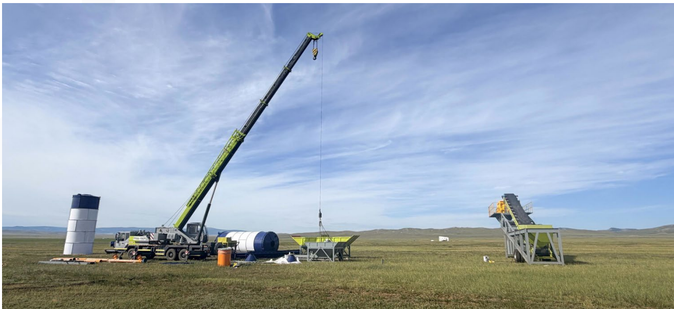
Figure 3. Unloading of concrete batching plant equipment following mobilisation to the CHPP site.
