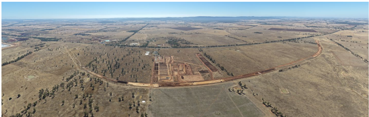
Newell Highway works looking east.
