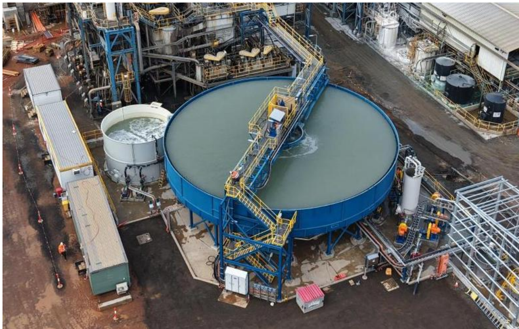
Figure 1. New 22m tailings thickener now in operation.
