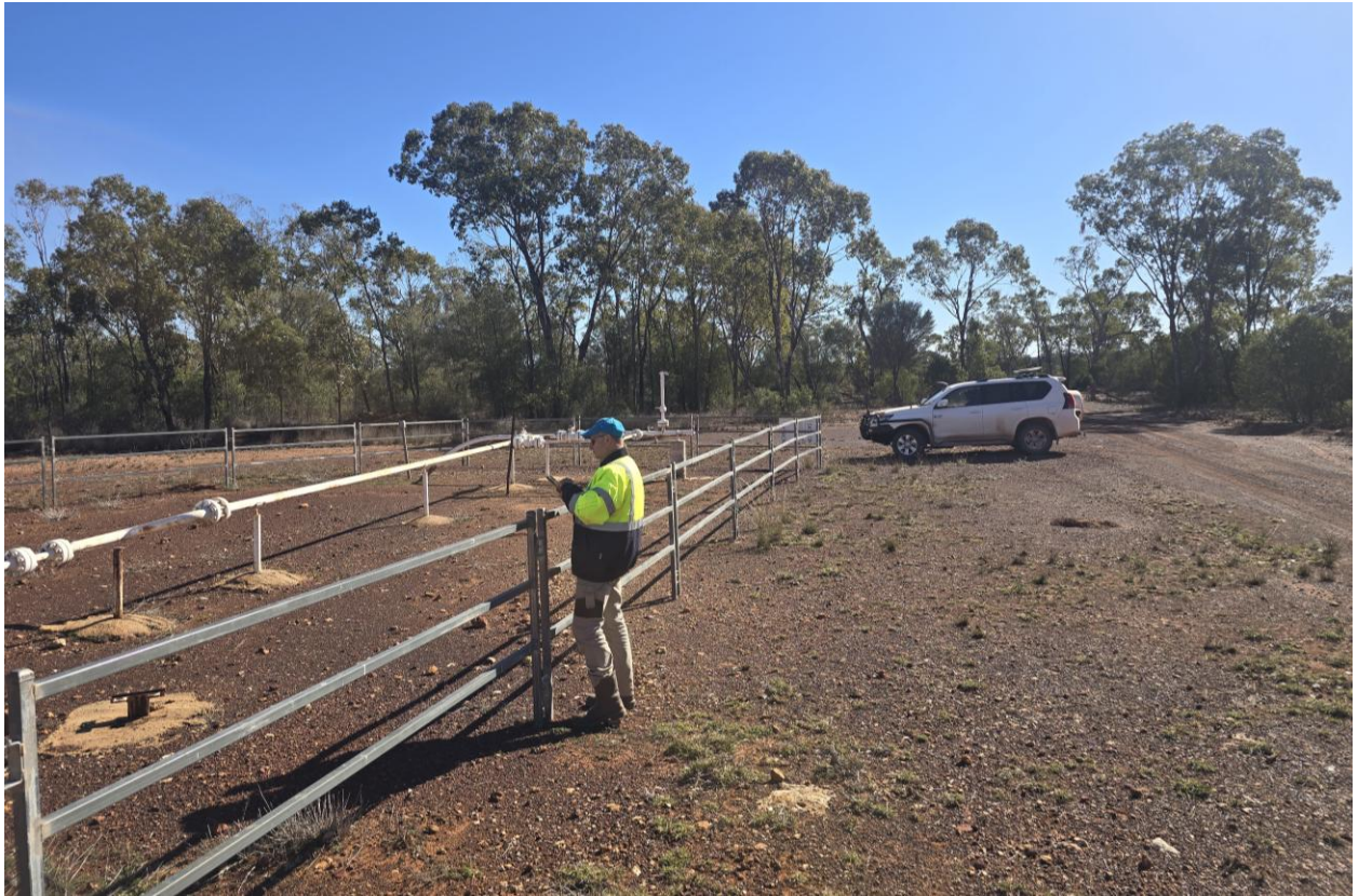
Figure 6 Boxley Pipeline Connection (white line section left to right) with Major connection and riser in background
