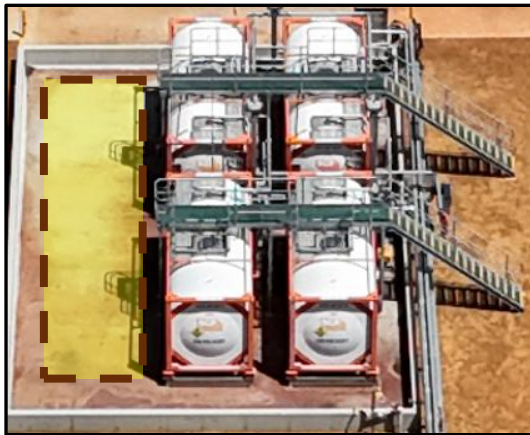
Raw Materials Storage Expansion
