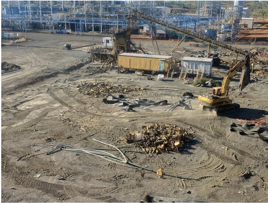
Image 2 - Crushing Circuit Demolition Commenced
