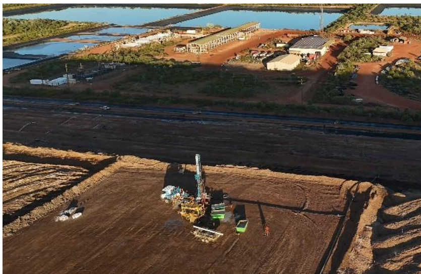
Image 1 - Installation of injection bore Pad 14 – Jex-Technology
