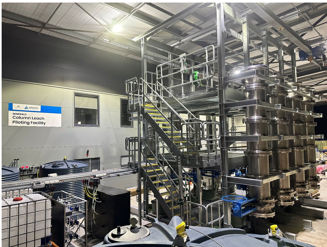
Figure 1 ANSTO column leach piloting facility
