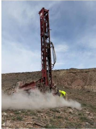
Figure 8: Aircore drilling rig at the Yellow Cat project.
