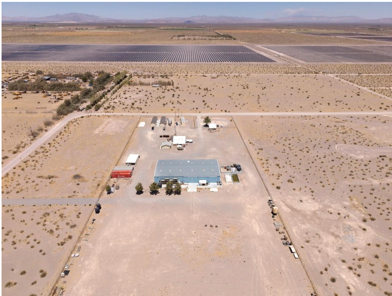
Figure 2: Aerial view of the Del Sol Refinery, with the neighbouring utility-scale solar farm visible in the background.
