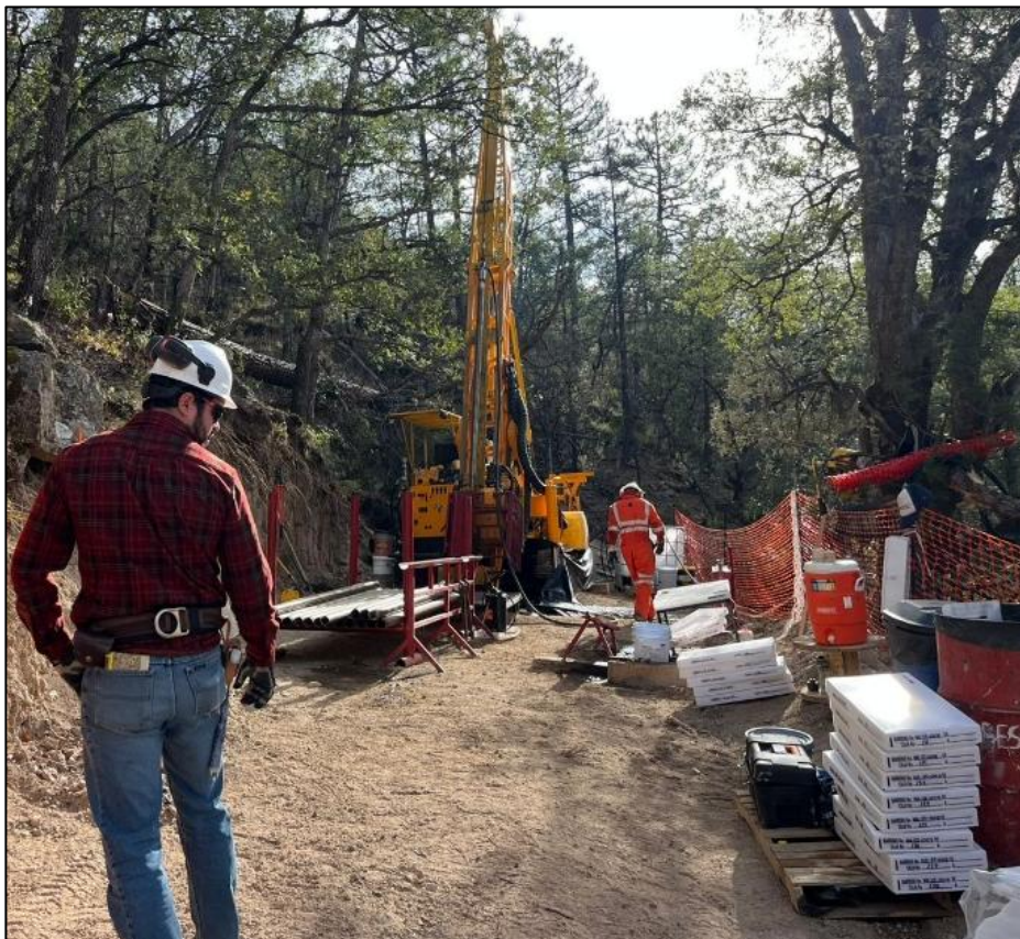
Figure 2. Photograph of the diamond rig set up and drilling hole YQ-25-009 in the central portion of Pertenencia at Yoquivo.
