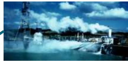
Pilot Plant Testing (C1 well, 1981-82)
