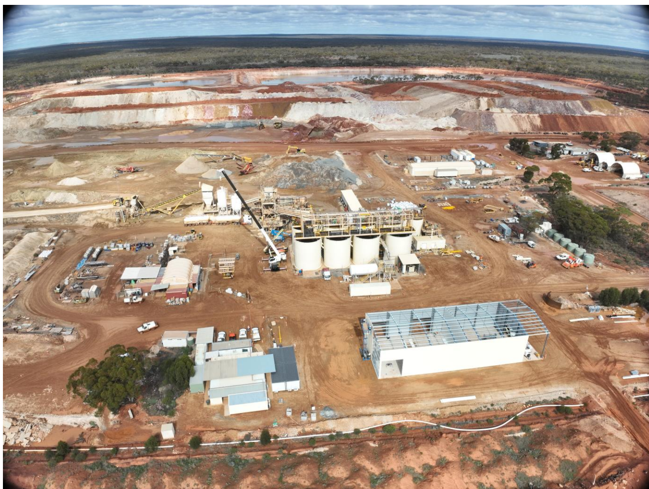
Image 3 – Jaurdi Gold Project Mill Upgrade – 28 July 2026
