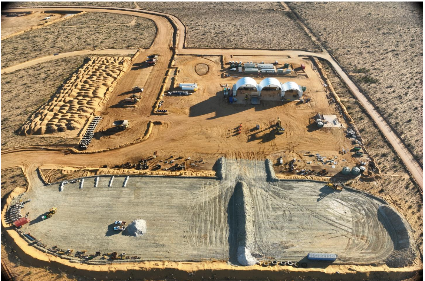
Image 2: Workshops, Offices and Infrastructure at Iguana 28 July 2026
