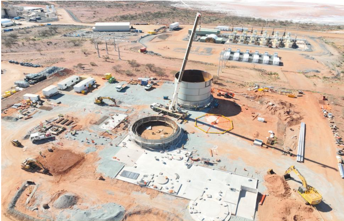
Paste plant Construction on 24 July 2026
