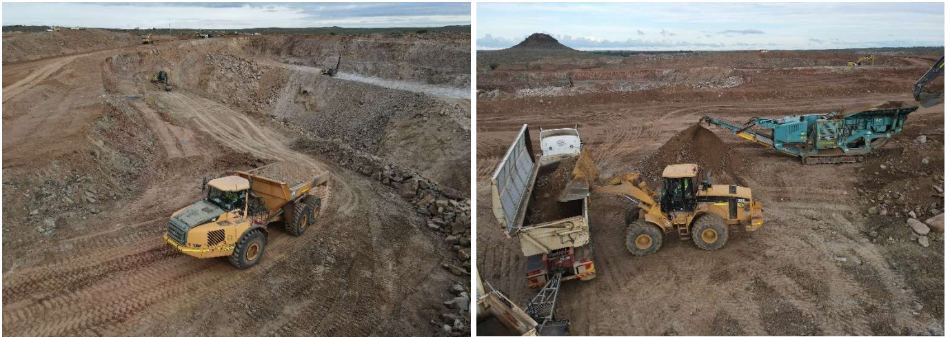
Figures 5 & 6 – Open Pit & ROM operations at the Pinnacles Mine with haul truck loading for transport to Rasp Mill
