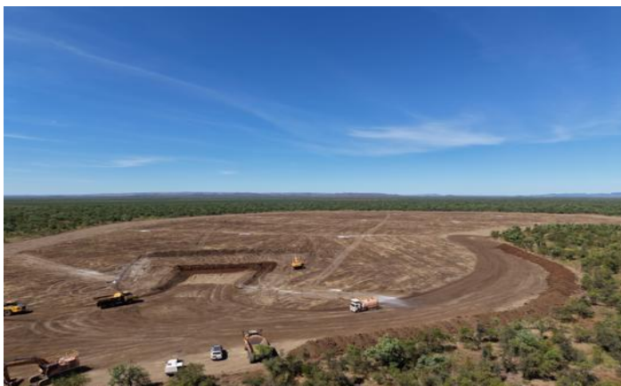
Figure 5: Excavation of B Pit
