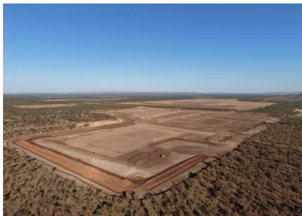
Figure 6: Evaporation Pond Construction
