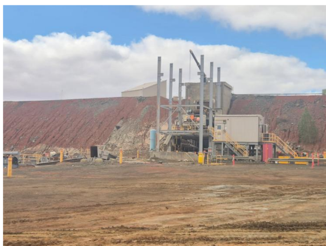
Figure 1: Primary Crusher Conveyor Removed
