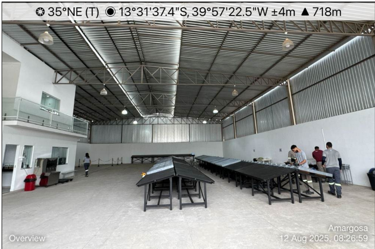
Figure 5-6: Amargosa logging facility
