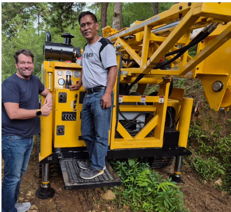
Figure 1: Blackstone's drill rig has arrived onsite
