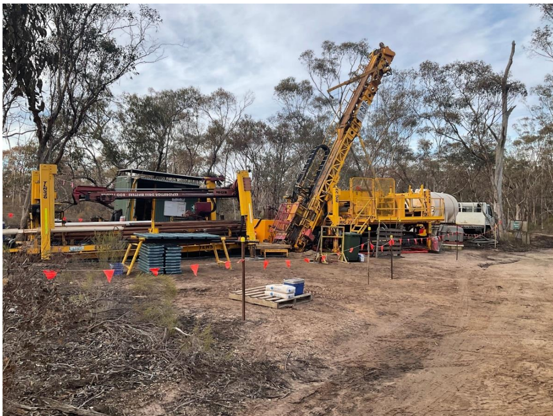
Figure 6. Drilling at Crosbie South.
