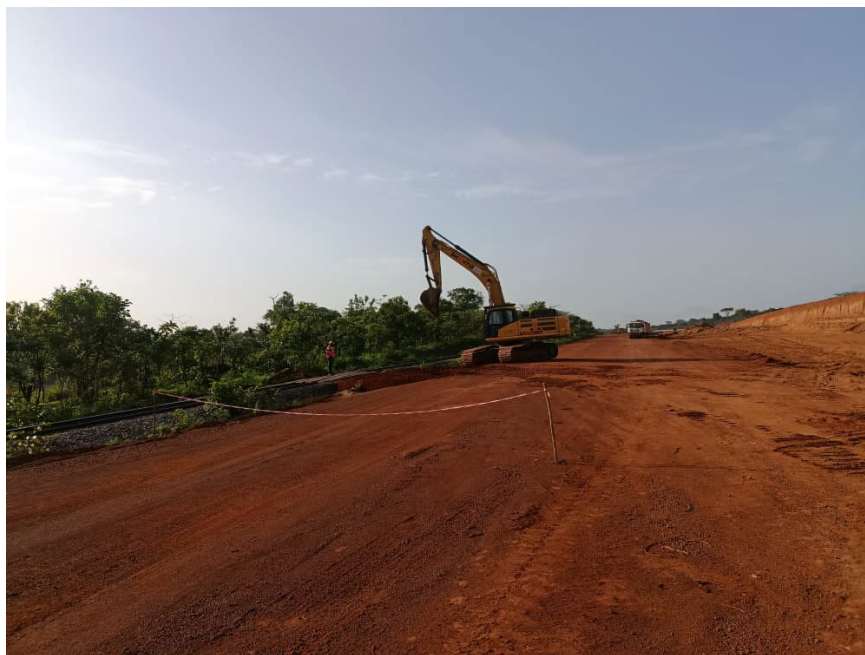
Image 6: Site works at IRF
