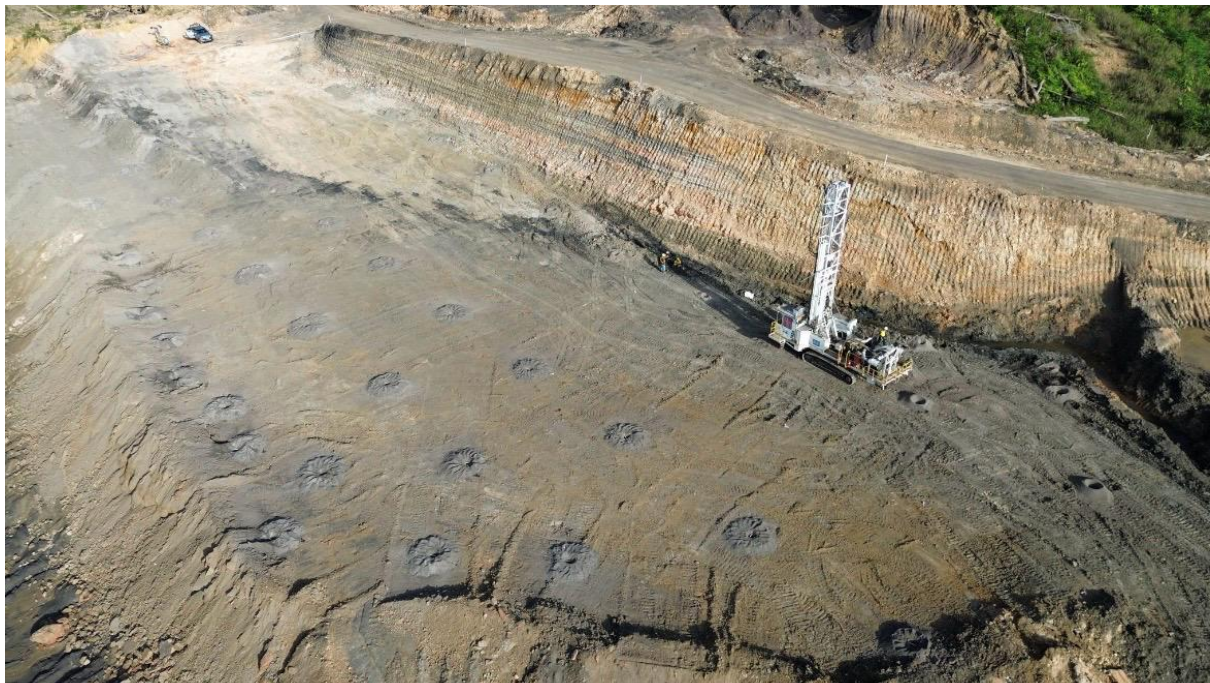
Drill and Blast Operations at Pit 3
