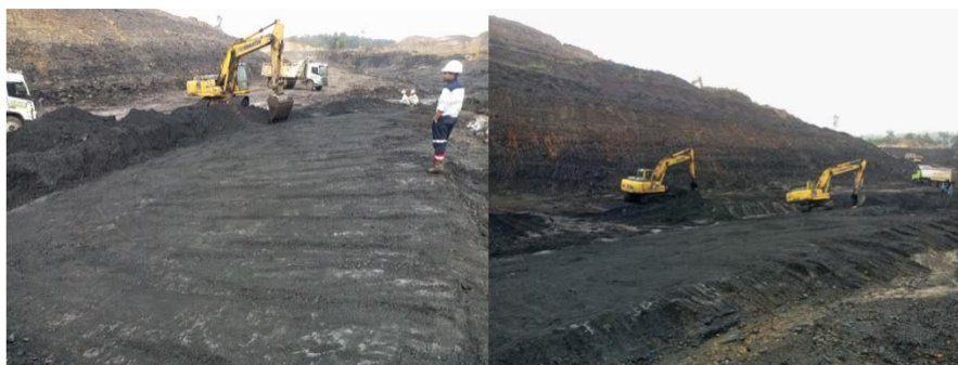
Mining Operations at Pit 3
