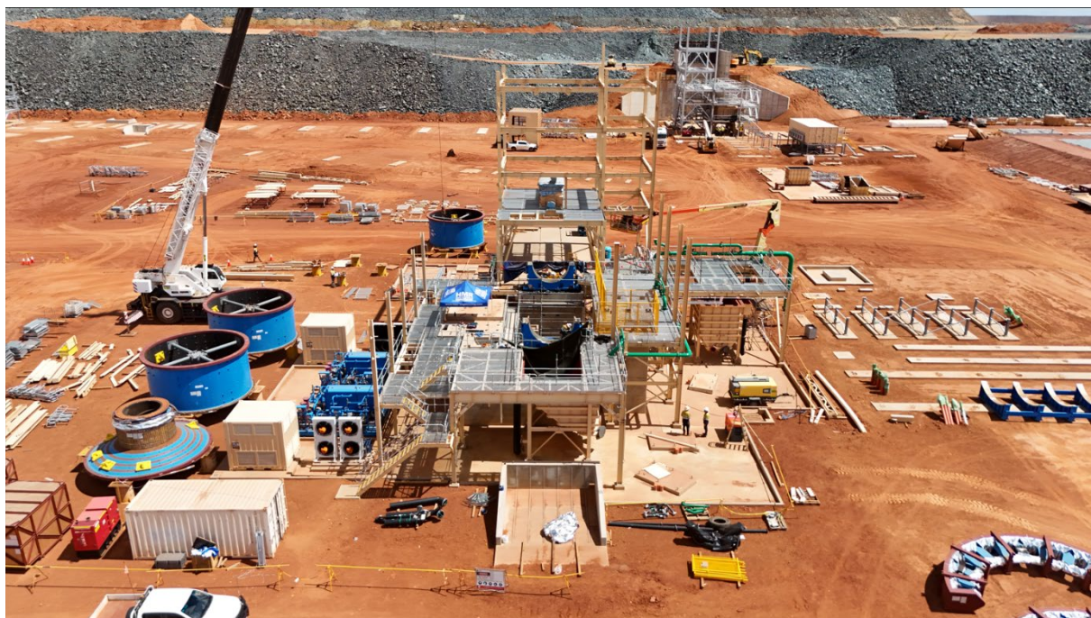
Karlawinda Expansion Project – Mill and crusher areas with mill sections being placed.
