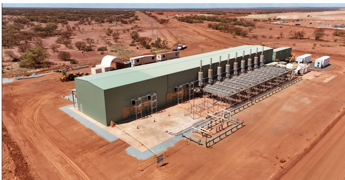
Karlawinda Expansion Project – Power station extension.
