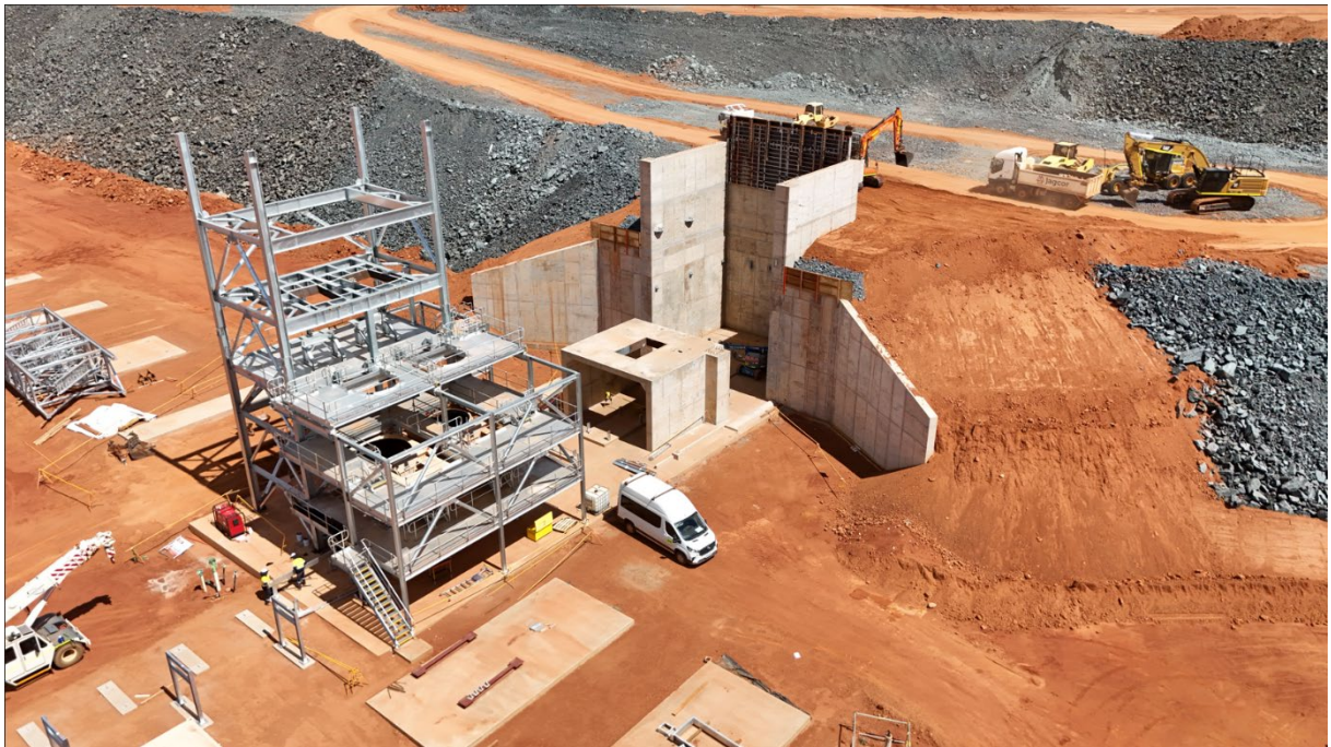
Karlawinda Expansion Project – Primary/Secondary/Tertiary crusher building and ROM 2 tie in.
