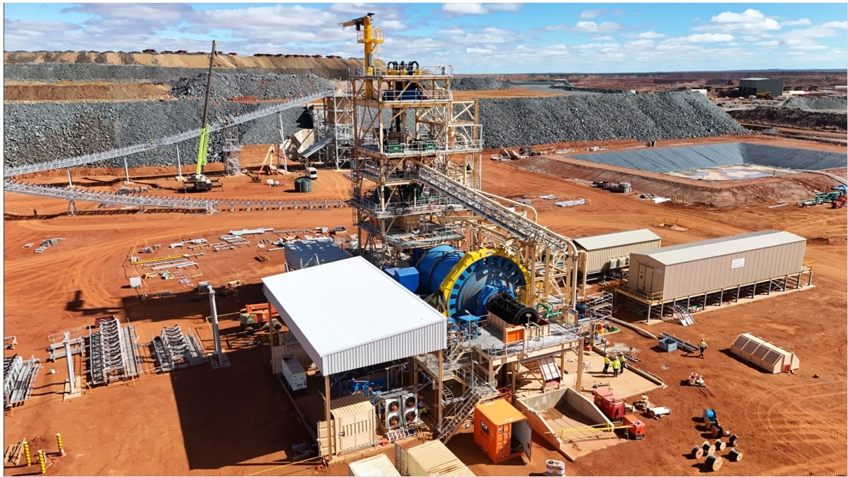
Mill area nearing completion.
