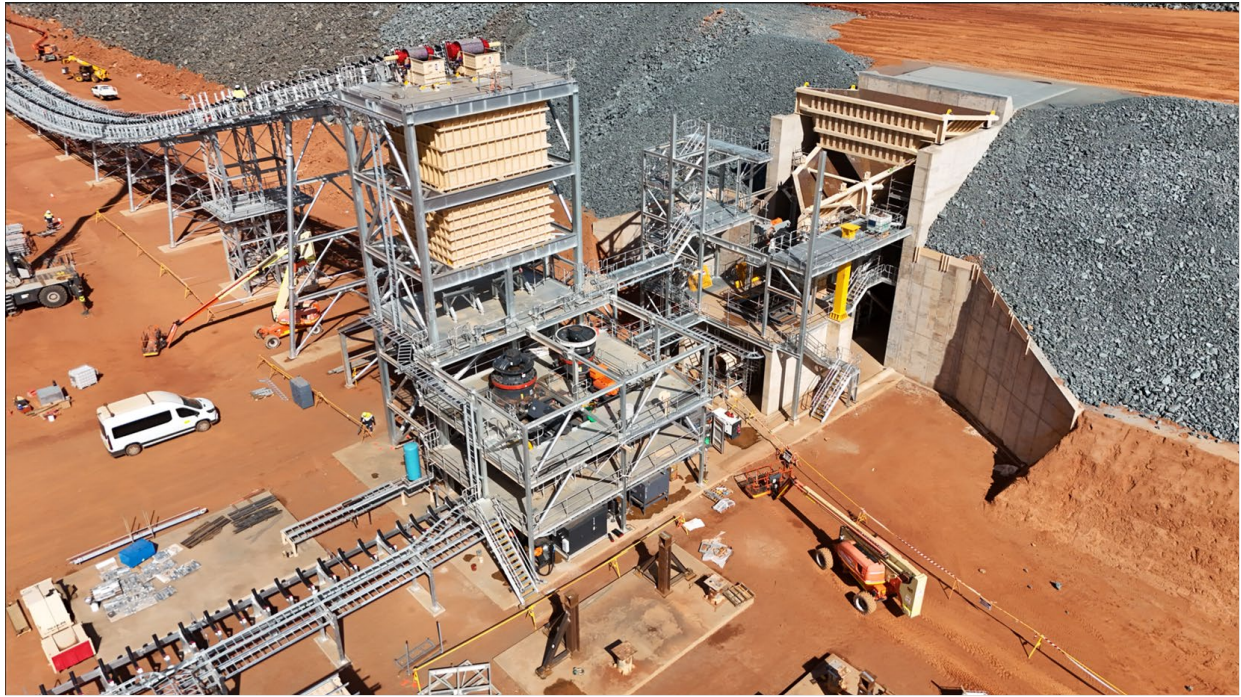
Primary/Secondary/Tertiary crusher building and ROM 2.
