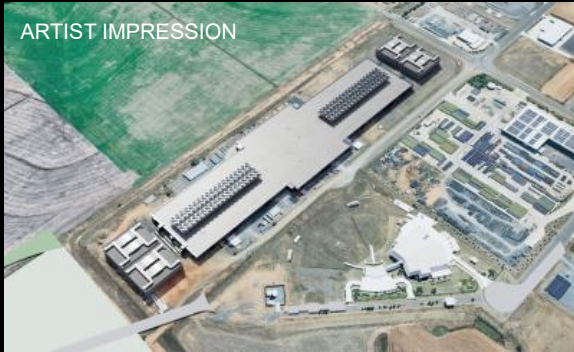
WELLCAMP TOOWOOMBA DC, EXPANSION
