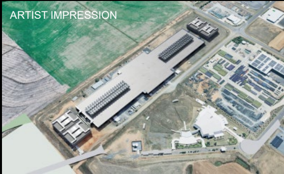
WELLCAMP TOOWOOMBA DC, EXPANSION
