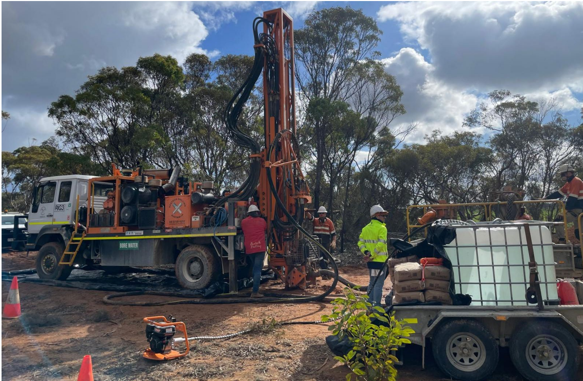
Figure 13: Drill rig mobilised at Cummins Project.
