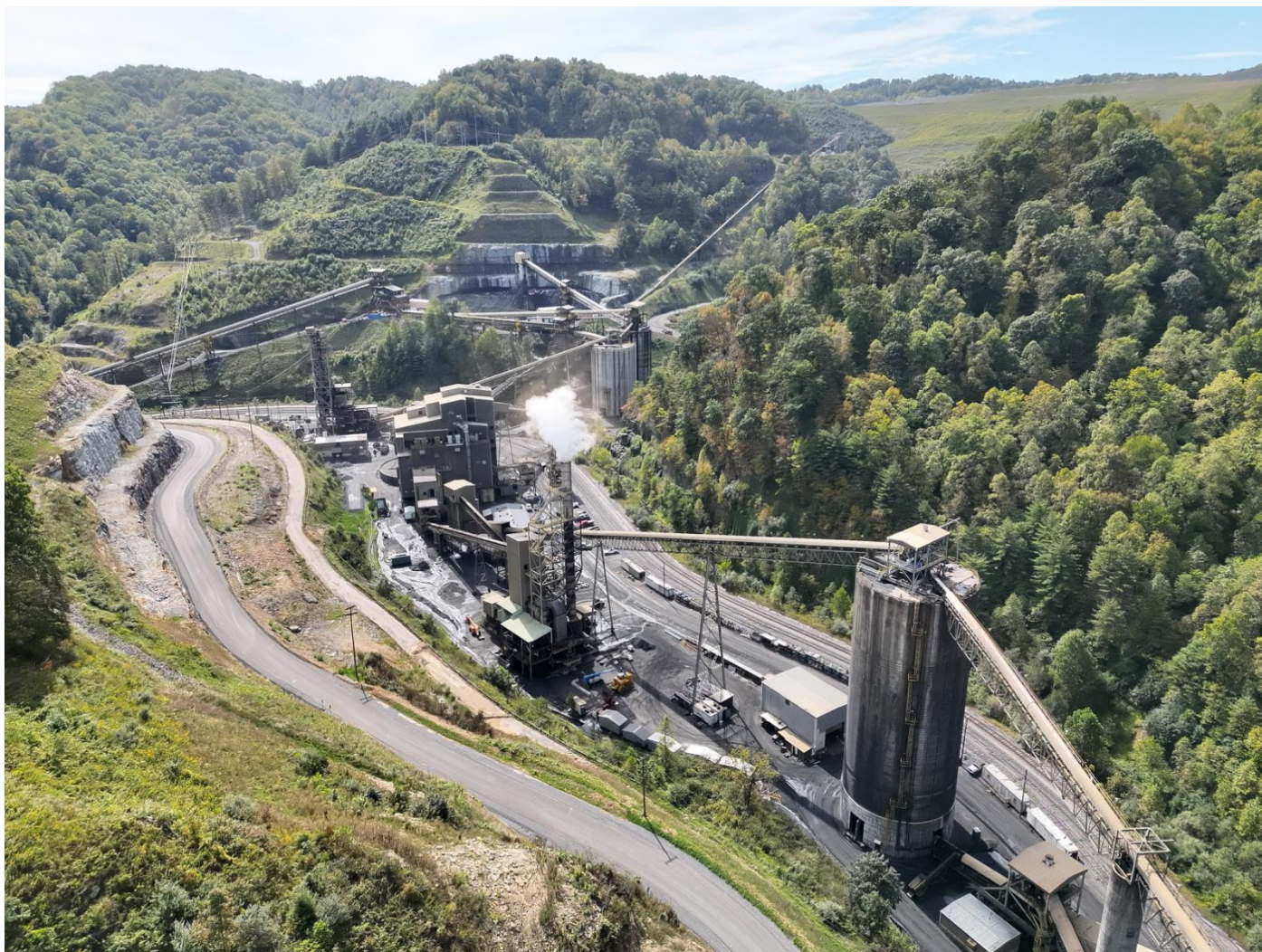
Buchanan Coal Handling and Processing Plant with Buchanan expansion complete.
