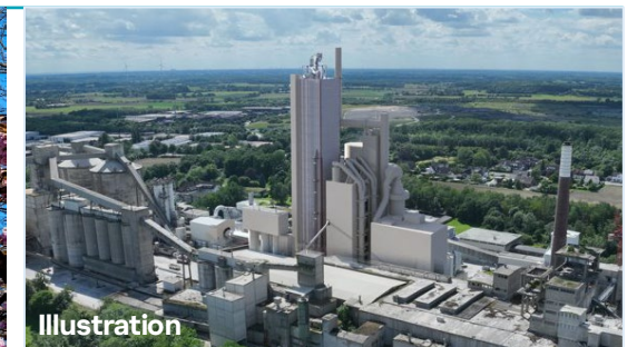
Leilac-2 demonstration plant for Heidelberg Materials cement plant – Ennigerloh, Germany
