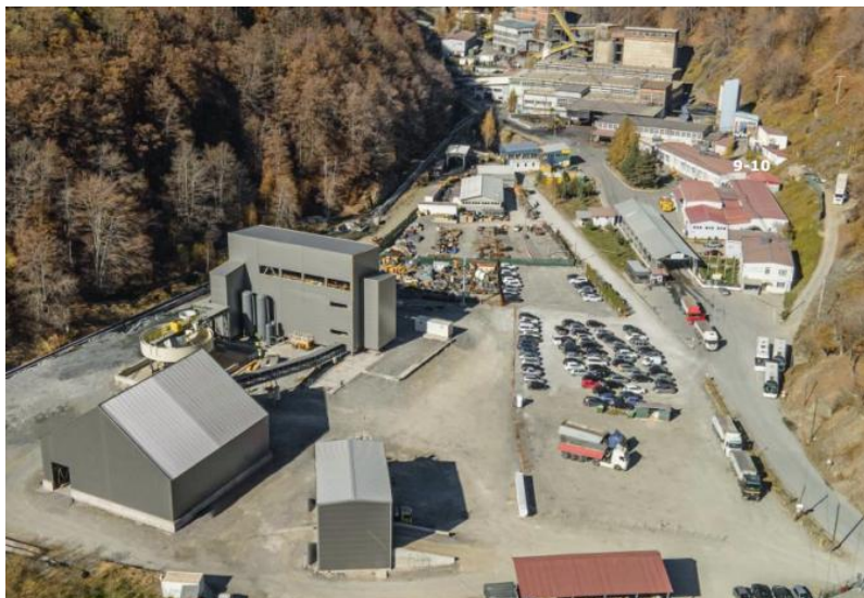
Figure 54 - Overview of the Sasa Project
