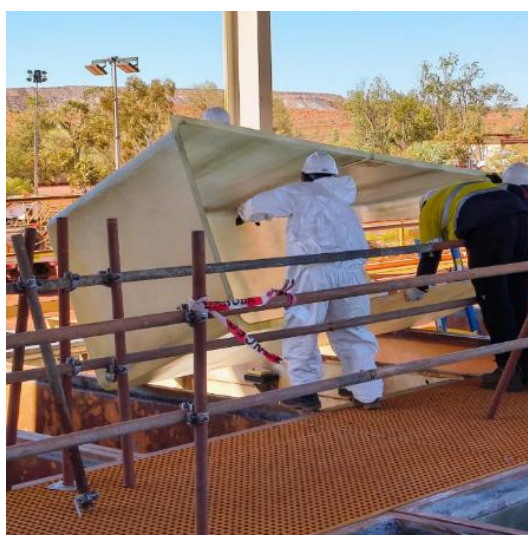
Installing fiberglass inserts for EW cells
