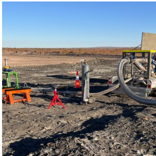
Testing direct injection leach system with water
