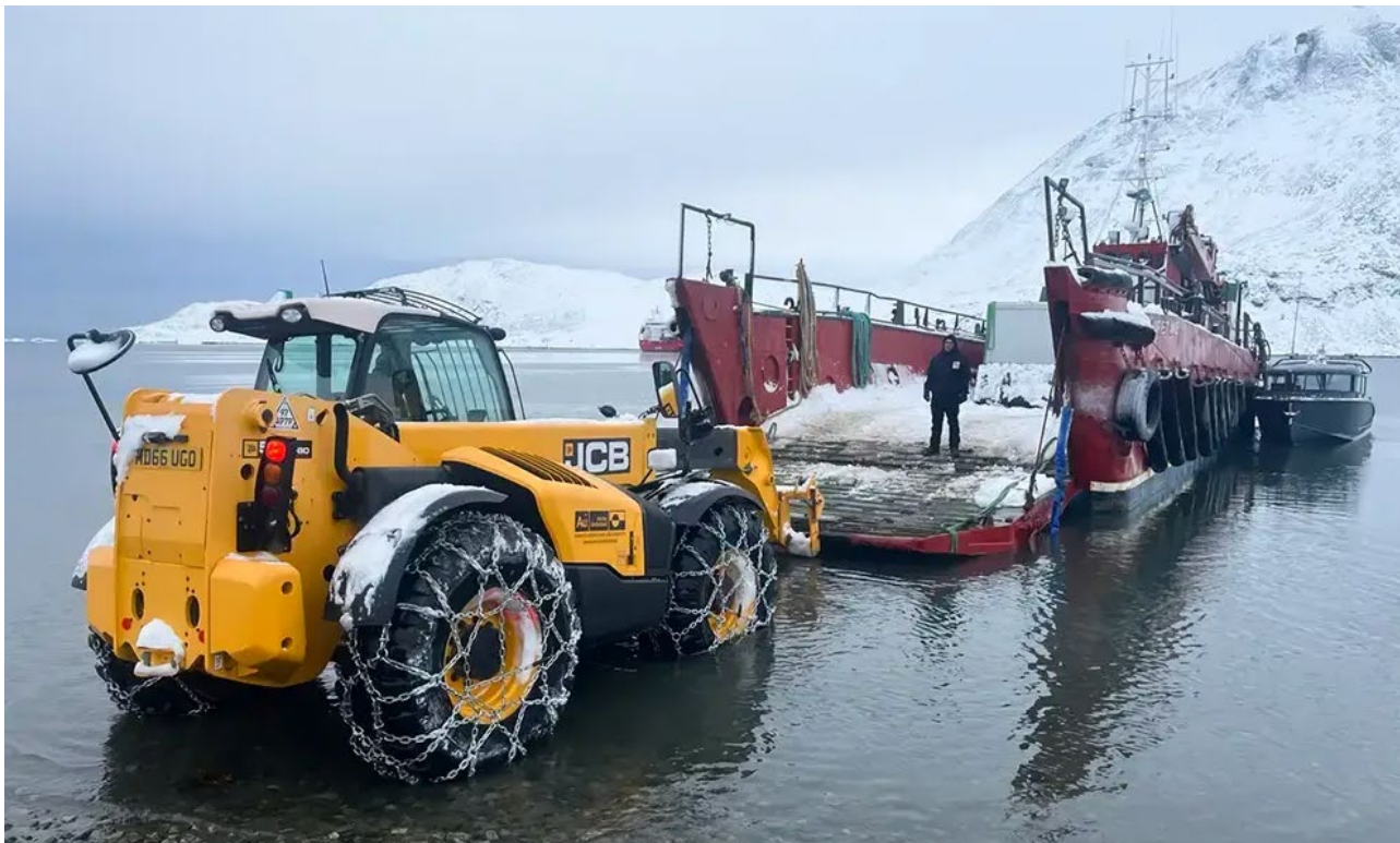
Figure 1. Barge and equipment being mobilised to site.
