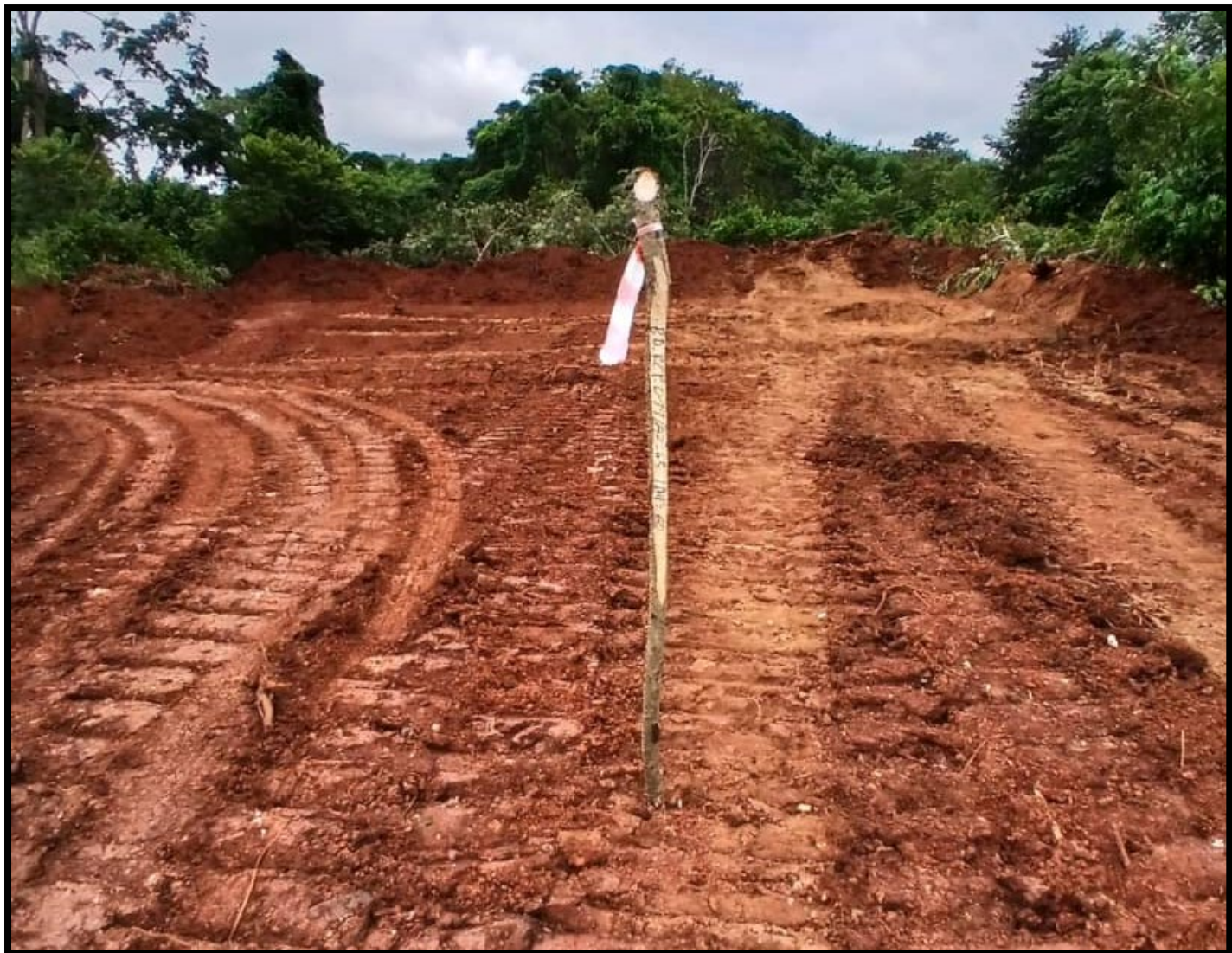
Figure 3. Drill pad preparation complete at Wilfred target.
