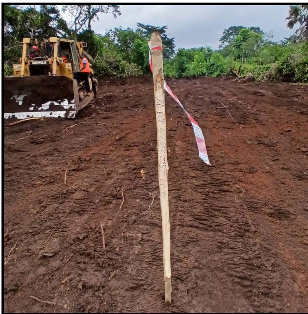
Figure 1. Initial drill pad preparation completed ahead of RC drilling at the Bondoukou Gold Ridge Project.
