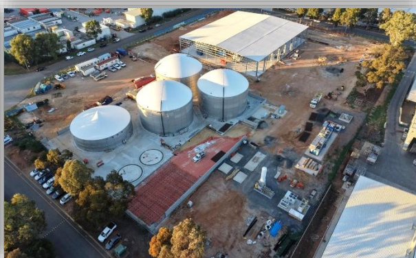
Image 7-9: SA1 Salisbury Bioenergy site works
