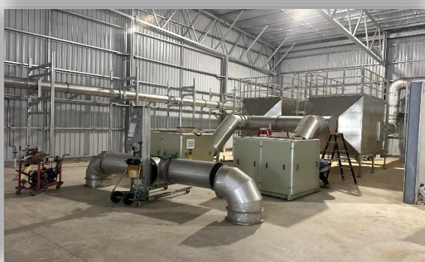
Image 2-4: SA1 Salisbury Bioenergy site works
