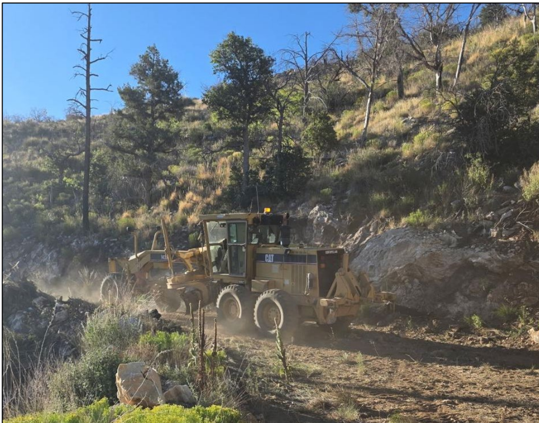
Figure 1 – Earthmoving equipment grading access road to drill site at Oracle Ridge
