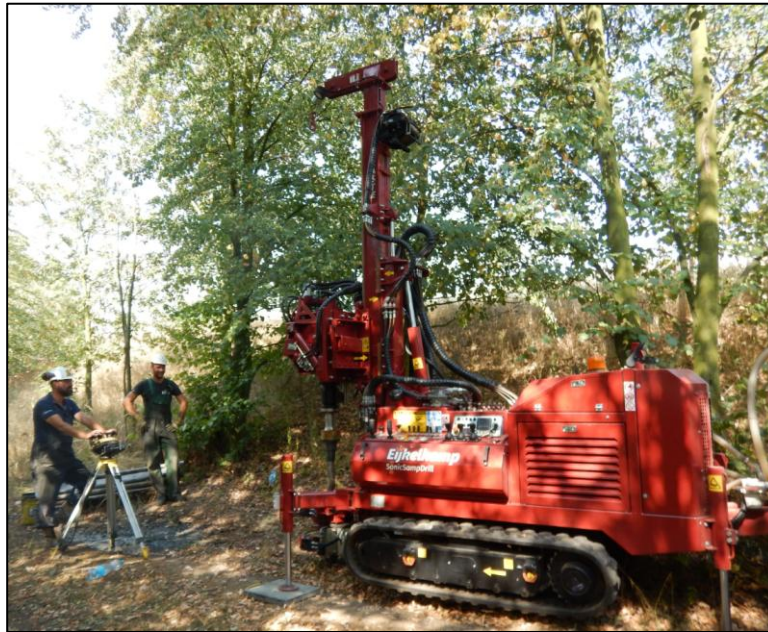
Figure 10-3: Eijkelpomp SonicSampDrill SRS Used for 2018 Sonic Drilling Investigation
