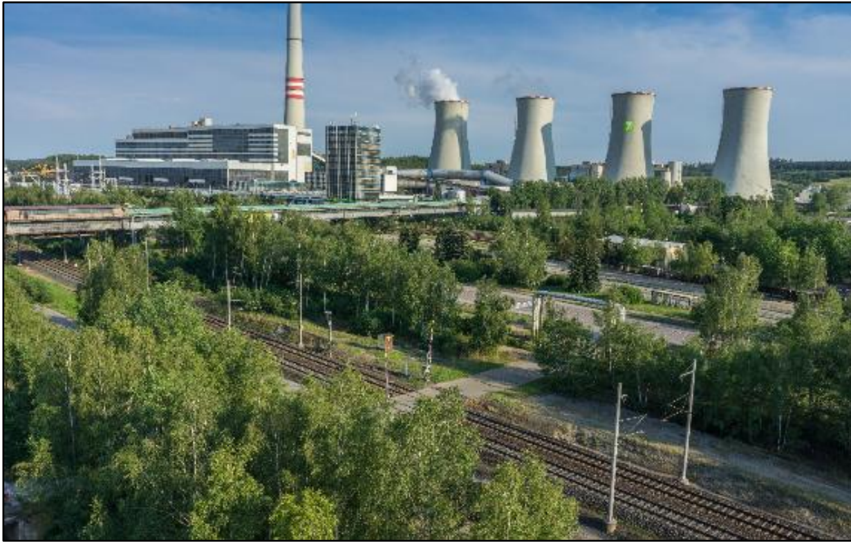
Figure 6-3: Current Power Plant
