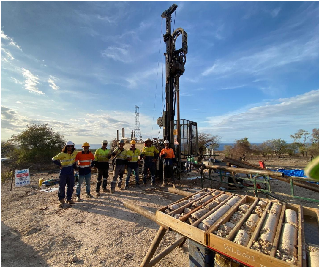
Figure 10: Collaring of the first diamond drillhole WLD001 at the Werumata Limestone Project with Estrella's exploration team and Coresearch drill team. 7
