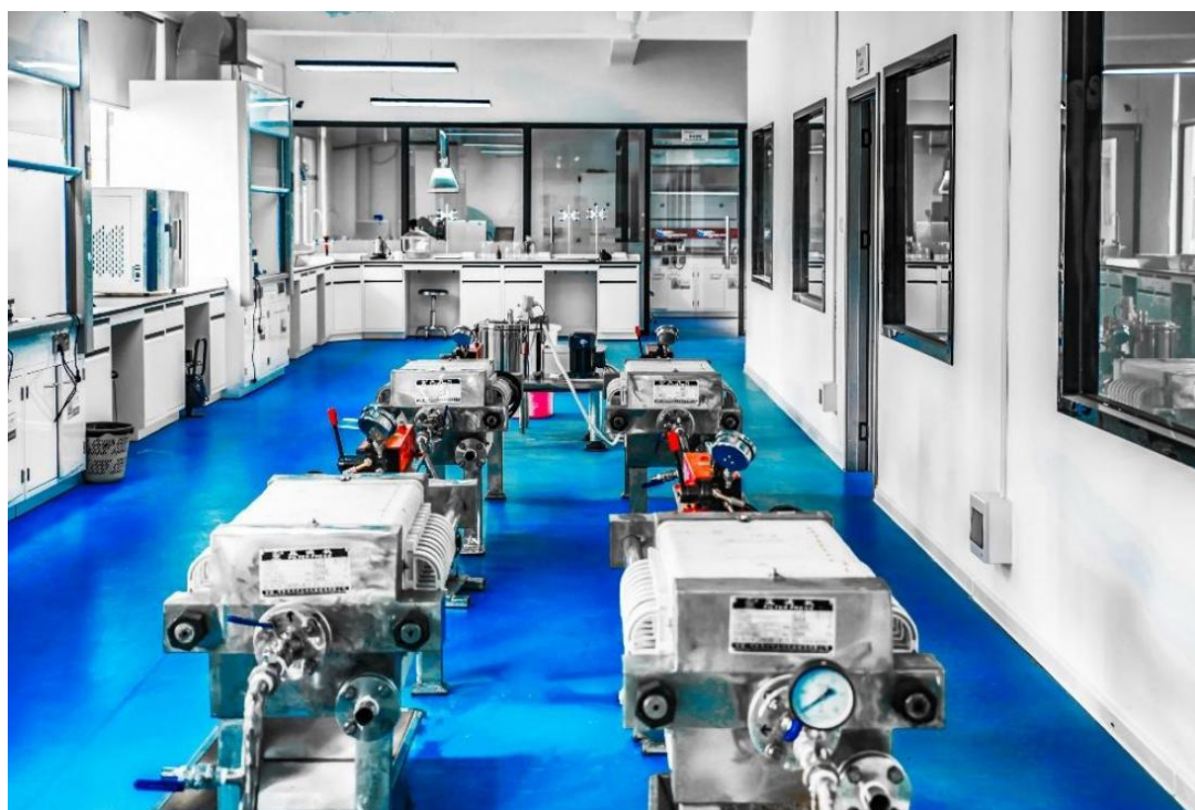
Figure 4: All key equipment for the ADP has been ordered, replicating a proven advanced manganese battery materials flowsheet from our China Pilot Plant.
