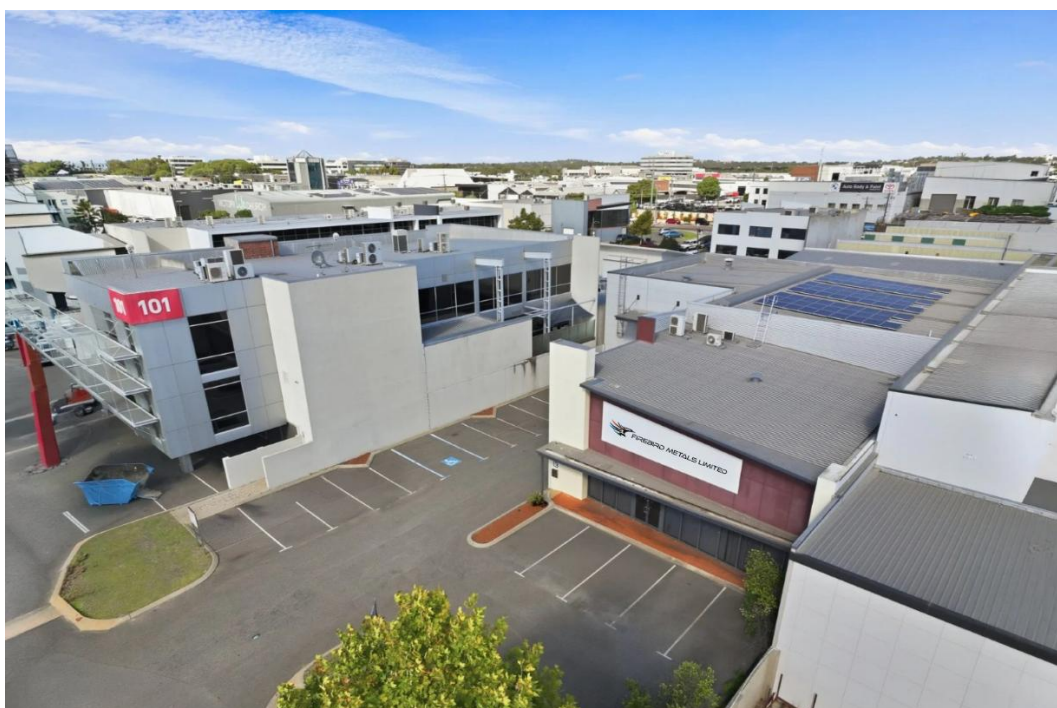
Figure 1: ADP property located in Osborne Park, Perth.
