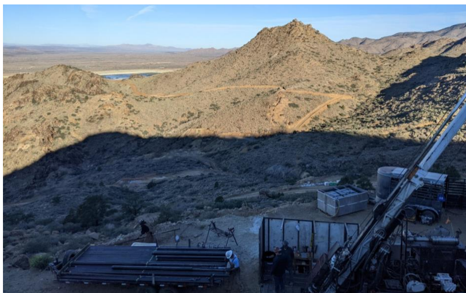
Figure 2 - Photo of core drilling in progress at Golconda (November 2025). Mineral Park in background
