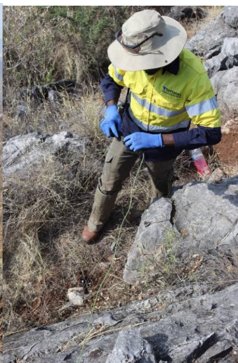
Image 5 : Connecting IP transmitter
