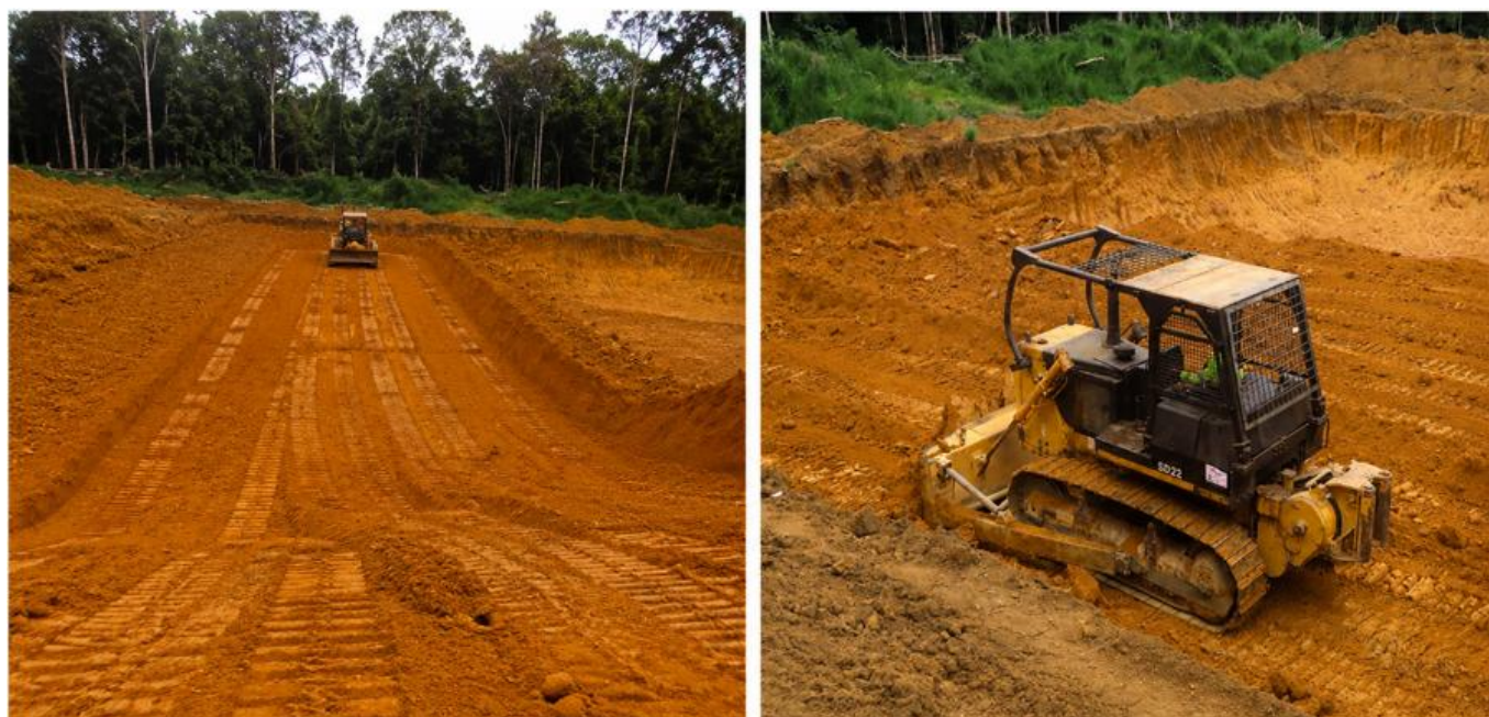
Figure 1 – Laterite Quarry – Overburden Removal.
