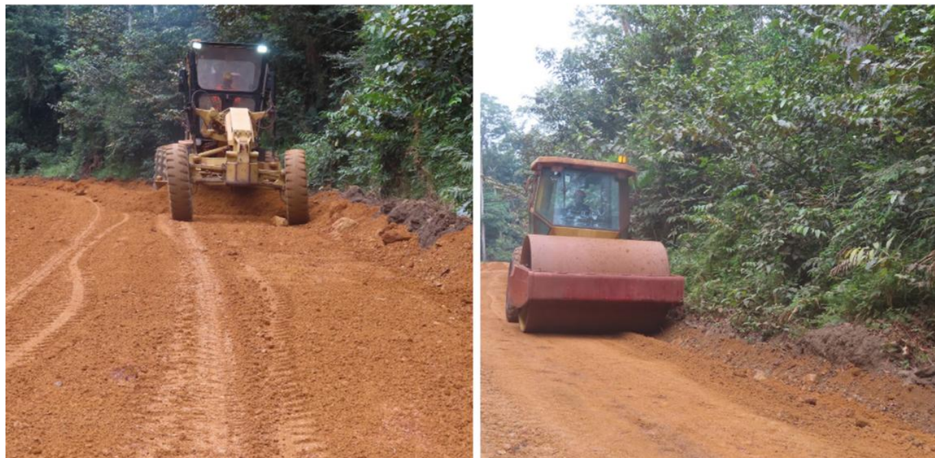
Figure 2 – Road Upgrades (Grading and Compaction)
