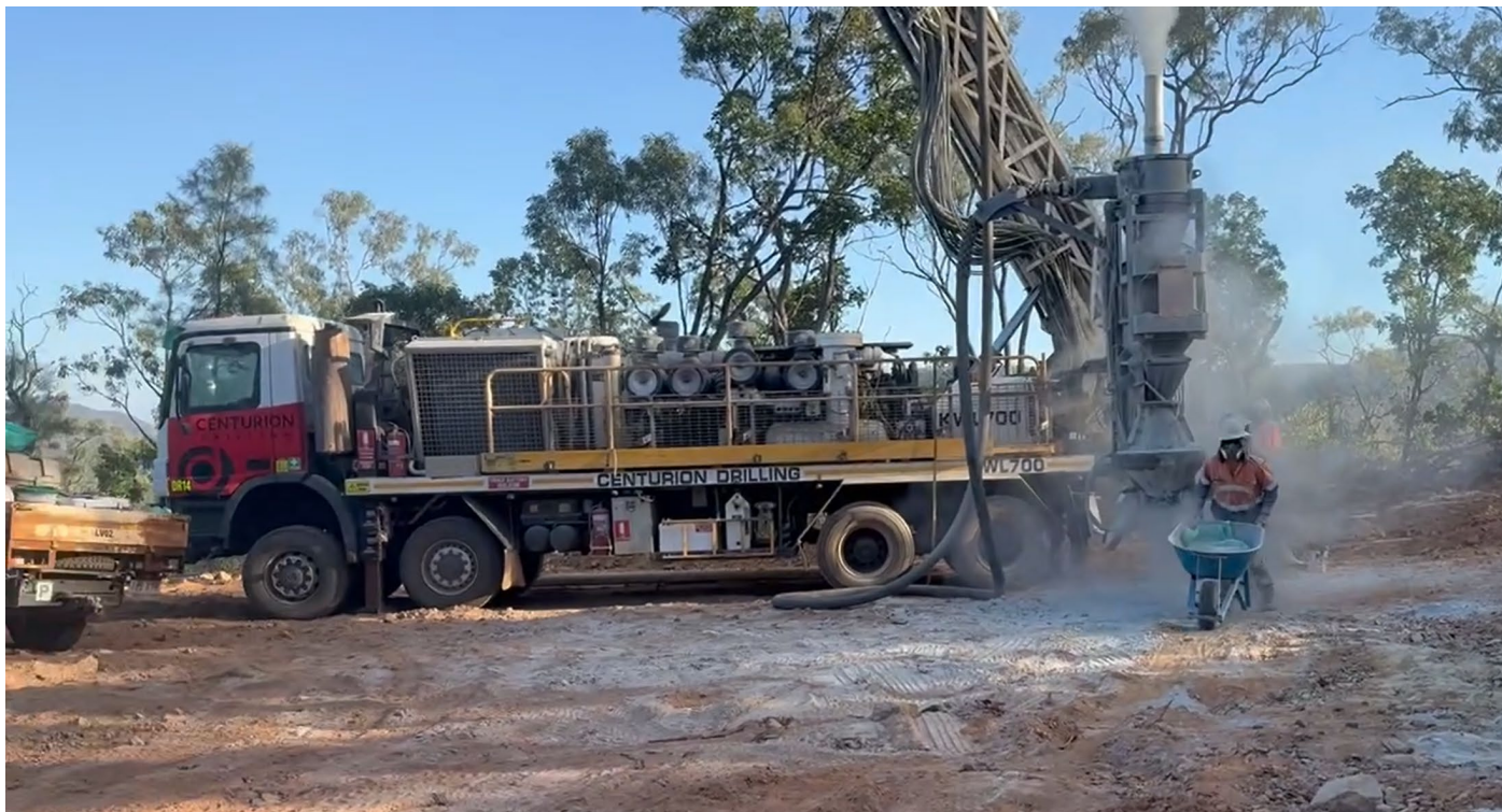
Figure 2 Drilling at Copper Hills in June 2026.
