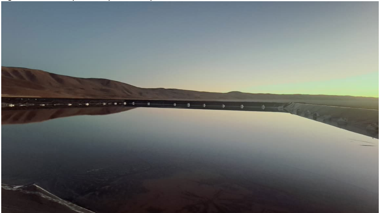
Figure 1. Final evaporation pond with processed brine.
