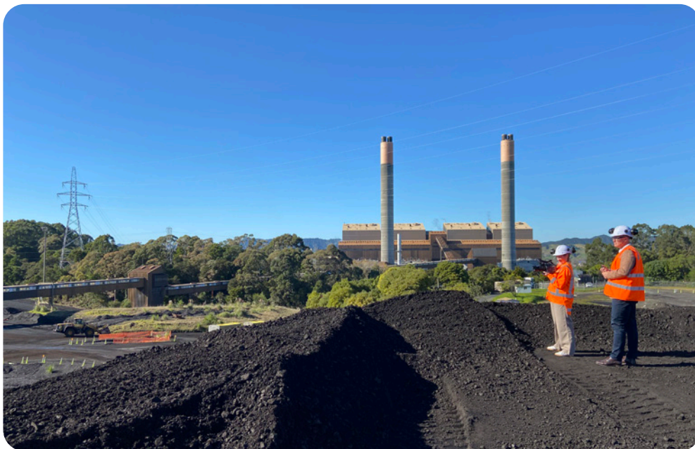
The coal stockpile at Huntly Power Station
