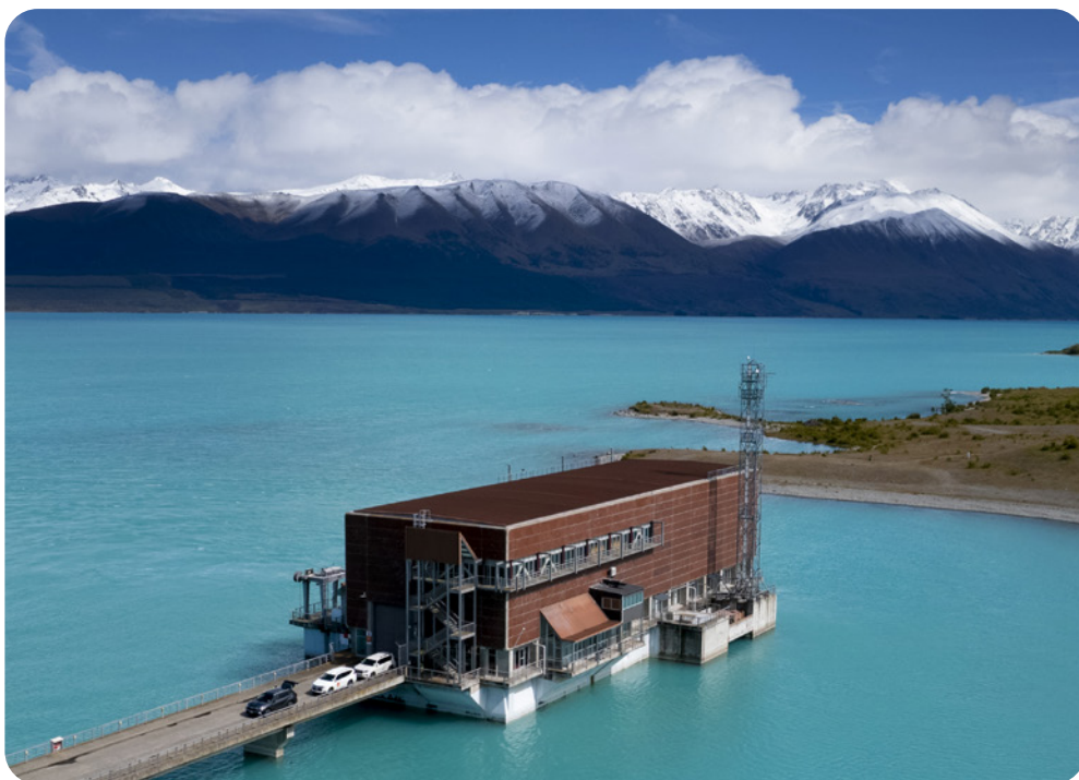
Tekapo B Power Station
