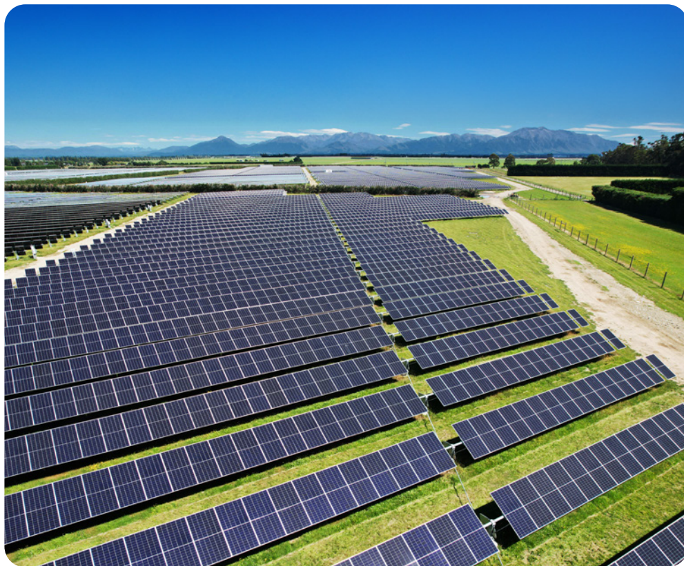
Lauriston Solar Farm
