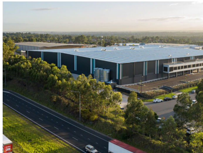
42 Cox Place, Glendenning, NSW
